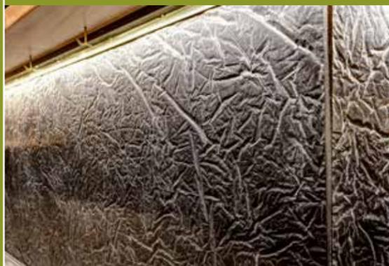
To create an organic texture on the front of the bar, Lujan and Blea "tried probably 100 different combinations of materials that we cast concrete against," before finally settling on a crinkled, shiny plastic that gave the concrete a unique textured quality. "We wanted it to be free-flowing, and to create shadow play and play up the light in the space," added Lujan.
