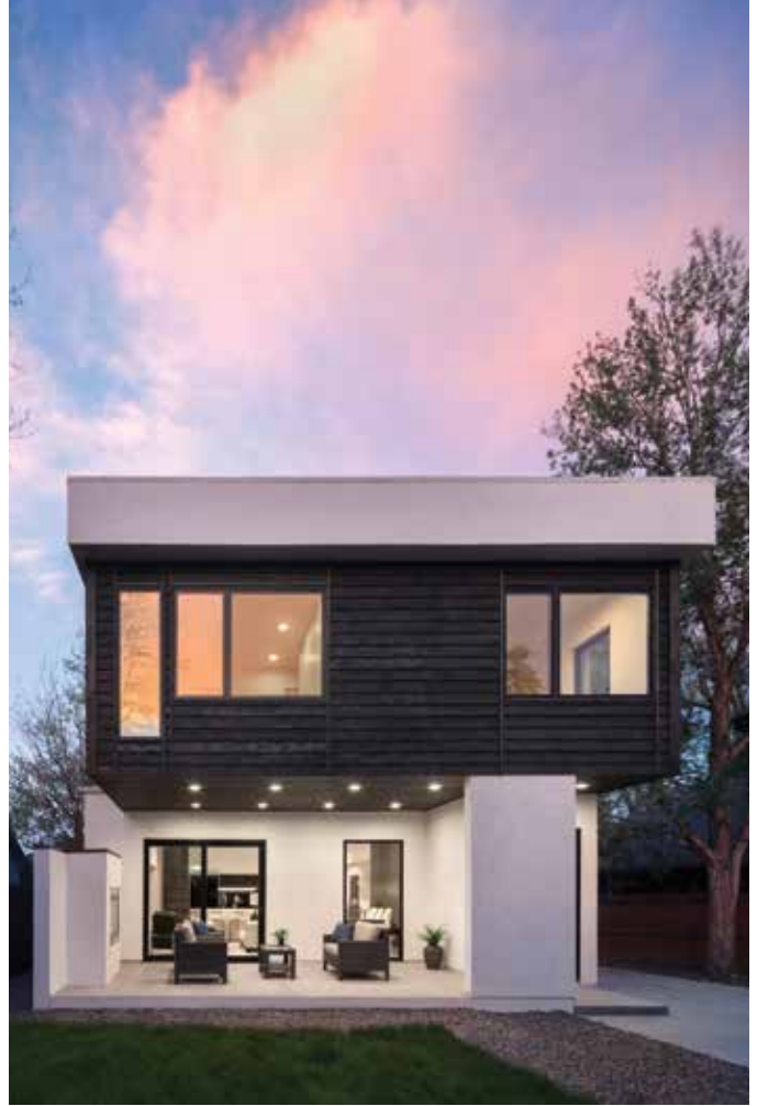
Architect Mitchell chose a Venetian plaster (opposite) for the non-pallet parts of the exterior; the material, made of limestone, has been around forever and leaves a surface that is ultra-smooth and shiny. For the home’s backyard (above) as well as the front yard, Mitchell designed rectilinear landscaping to reinforce the bold lines of the house. Bottom left, the home before its remodel.
