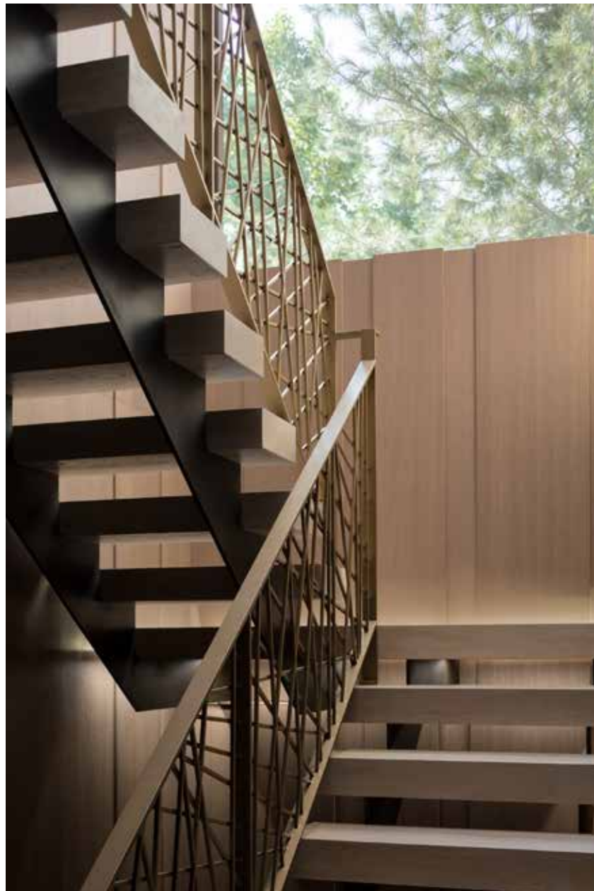
The custom staircase that connects the main floor to the basement level was designed by Blank to also appear to be floating. “I didn’t want to see a big ugly riser supporting the stairs, so every tread floats off of the walls.” He chose a brass custom railing to play off of the Lindsey Adelman chandelier in the dining room. “Everything feels right,” he says. “Your eye is not arrested anywhere. Everything just has this natural organic flow to it.”
